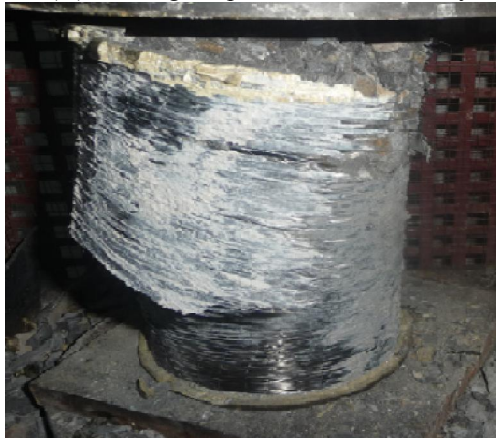
Fig. 1 (B) Rupture of cylinder wrapped with FRP
