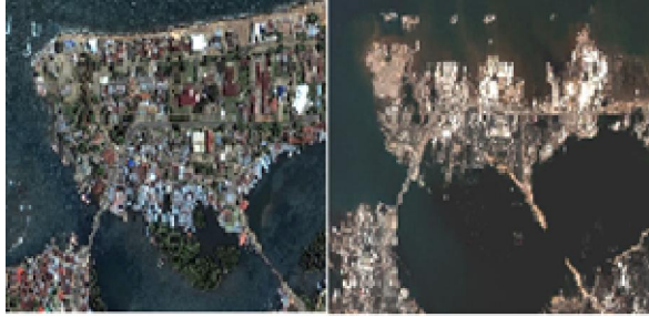
Figure 1. Effects of tsunami 2004, along coastal line and bridge structures in Banda Aceh, Indonesia.
