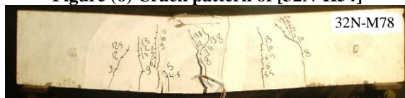
Figure (7) Crack pattern of [32N-M78]
