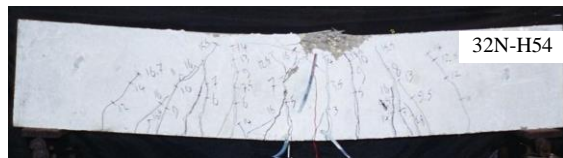
Figure (6) Crack pattern of [32N-H54]
