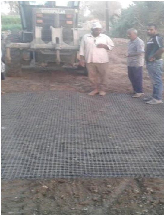
Fig., (3) reinforcing soil by geogrid in field.
