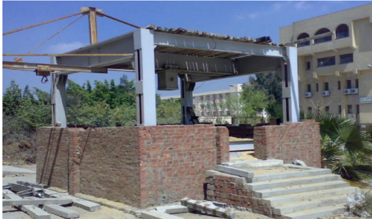
Fig (7) Soil chamber and loading frame
