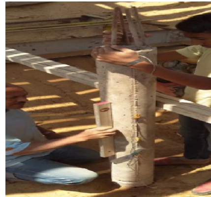
Fig (10) Alignment of pile - group (1)
