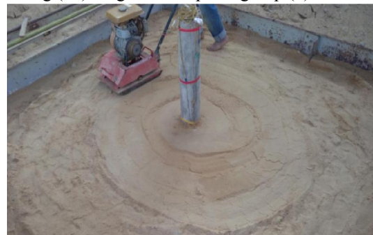
Fig (11) Placing compacted soil around tested pile for single pile- group (1)
