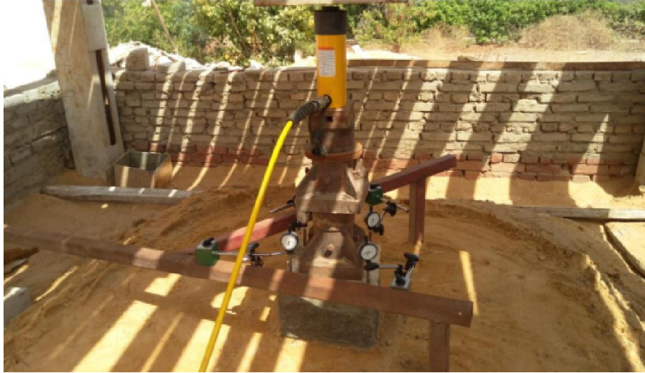
Fig (12) Reference beams and dial gauges setup for single pile- group (1)
