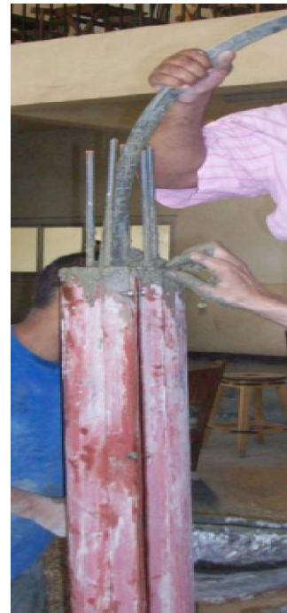
Fig (6) Casting of pile
