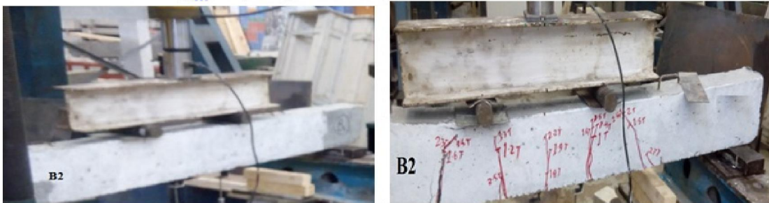
Fig. (22). Crack pattern of (B2) after burning at 400°C for 2 hours
