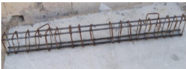
Fig. (17) Reinforcement was installed inside the beam mold
