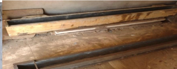
Fig. (17) Reinforcement was installed inside the beam mold
