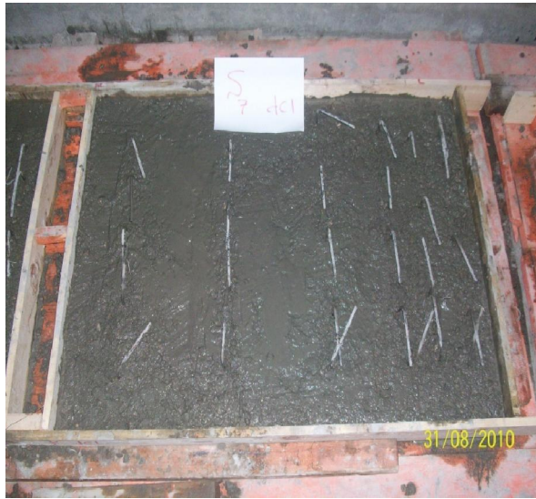
Figure (1): Pre-slab before casting the second layer.
