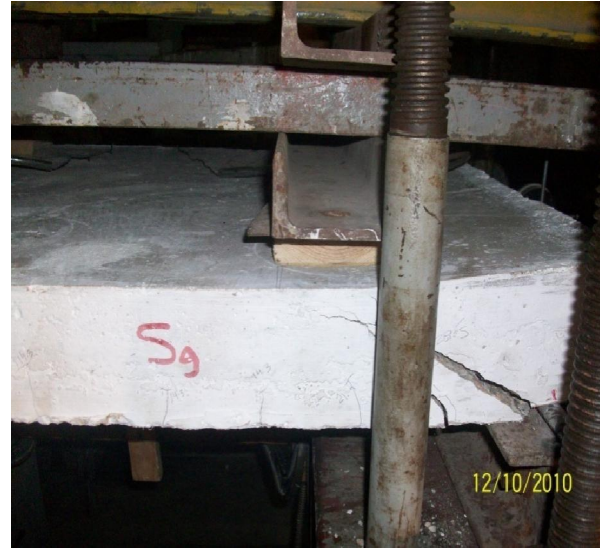
Figure (12): Shear failure of pre-slab S9.
