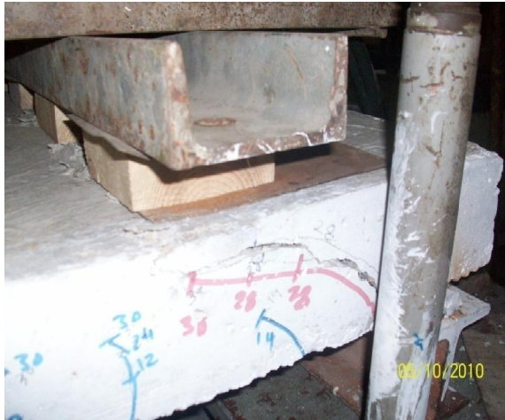
Figure (6): Shear failure of slab S3
