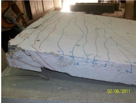
Figure (10): Shear failure of pre-slab S7
